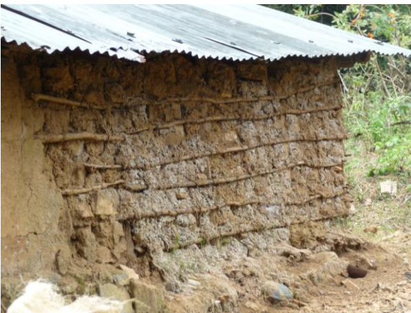
Left – the rebuilt kitchen wall
